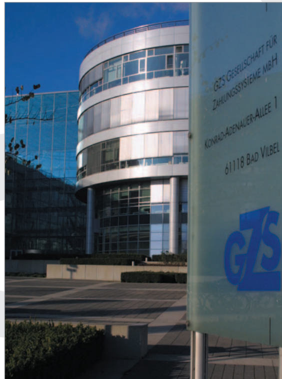
Central building of GZS in Bad Vilbel
